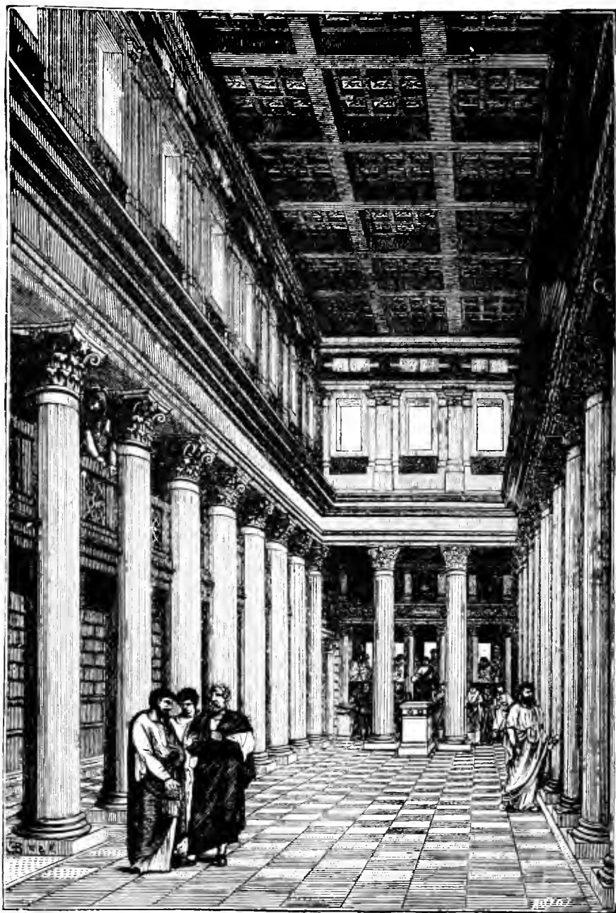
FIG 156.—INTERIOR OF A BASILICA AT POMPEII.
